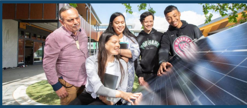
Figure 1 Solar panels installed by the partnerships. Photograph permission received from the school.
